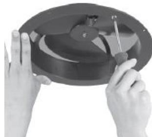
**Fig. 2 – Tightening mounting screws**
